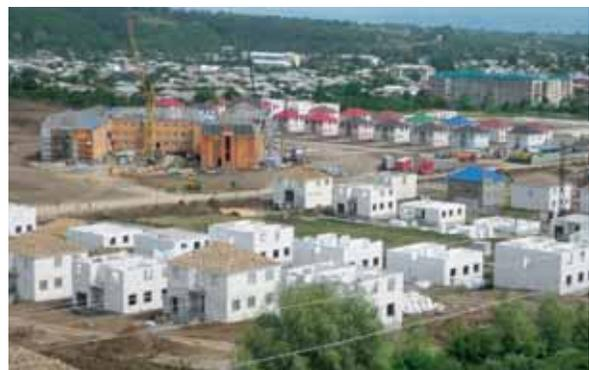
Picture 5 – Housing area during construction: production of all ICF elements with HEITZ Technology (in the back ICF houses already completed).
