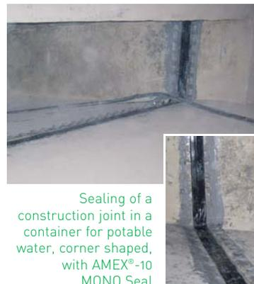
Sealing of a construction joint in a container for potable water, corner shaped, with AMEX®-10 MONO Seal
