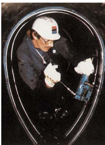
Installation of AMEX®-10 MONO Seal in an egg shaped sewer
