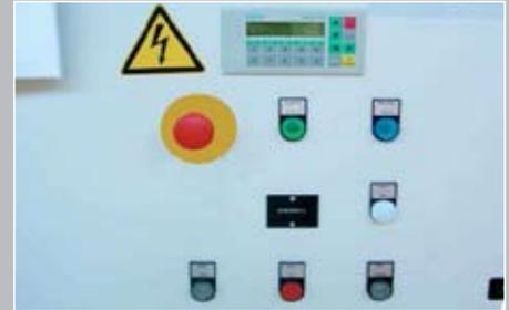
Stored-program controller PLC, operator panel with display.
