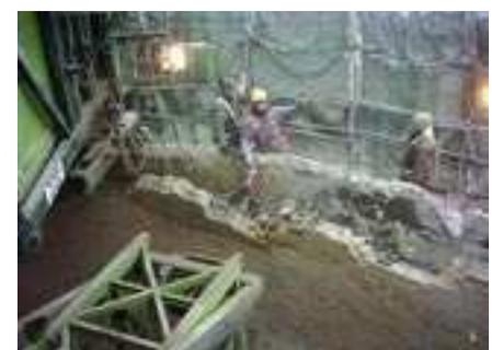
For the demolition of an industrial chimney the inner wall was systematically dismantled using a LUKAS spreader. The demolition of the chimney could not be completed using conventional methods as a blast at this location was not possible.
