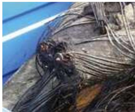
After being lifted from the ocean bottom the old ocean cables are shortened with LUKAS cutters so that they can be loaded for transport in containers.
