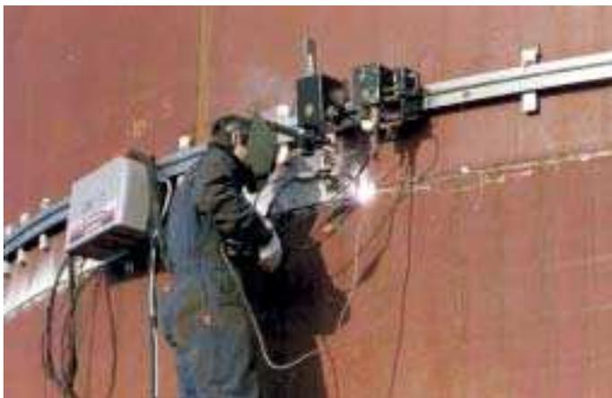
Aluminum Semi-Flex Rail (AFR) for large diameter applications down to a minimum radius of 15' (5 m). (Page 4)
