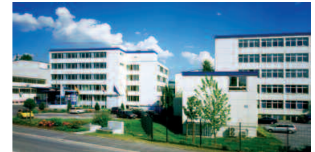
Dieffenbacher headquarters, Eppingen, Germany
